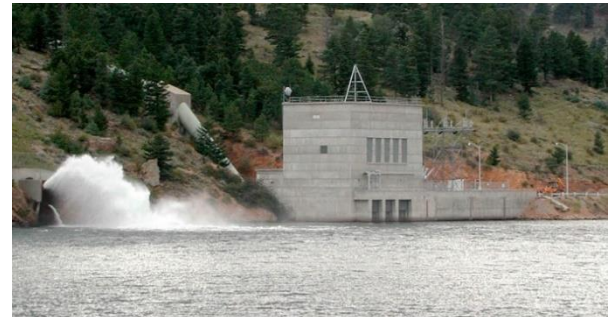
Mary's Lake Power Plant
