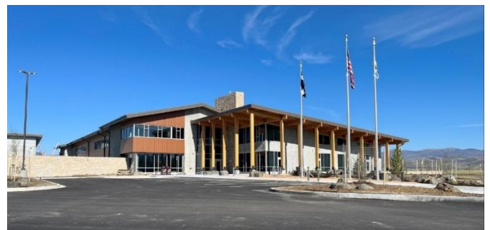
Northern Water opened its new Willow Creek Campus in Granby in September 2022. On the East Slope, Phase II construction began on a new wing for the main administration building.
