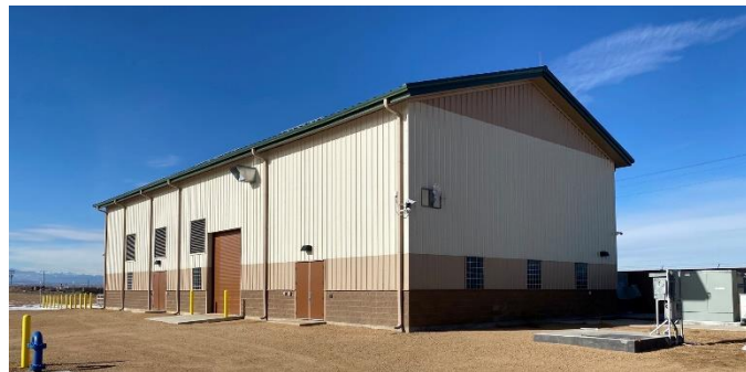
Eastern Pump Plant
