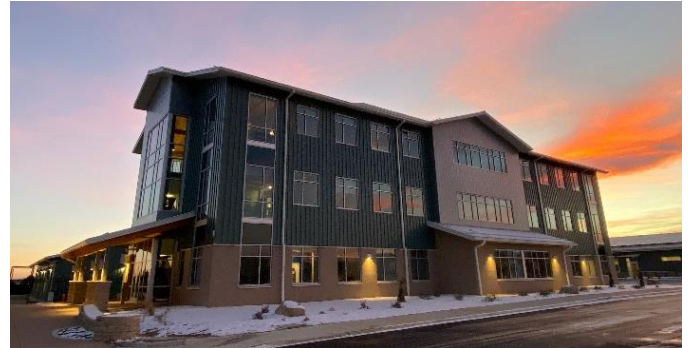
Phase I on the Berthoud campus included the new operations building which opened in the fall of 2022.
